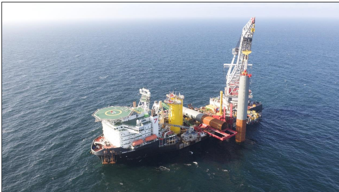
Figure 4.21: Monopile Installation (Photo courtesy of Dogger Bank Windfarm)
