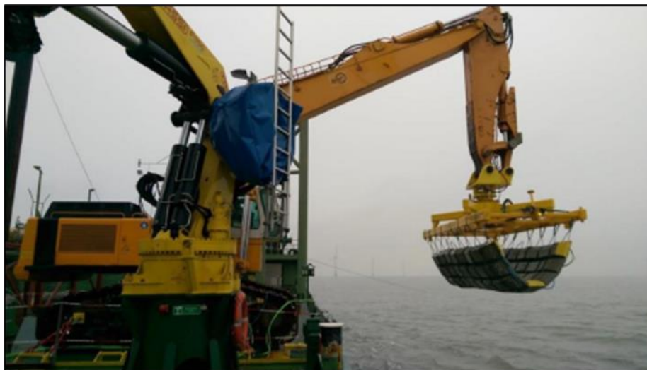
Figure 4.15: Concrete mattressing
