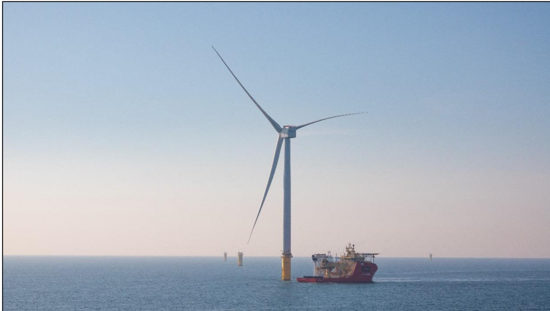
Figure 4.23: Installed offshore WTG with Monopile and TP installations in background (Photo courtesy of Dogger Bank Windfarm)
