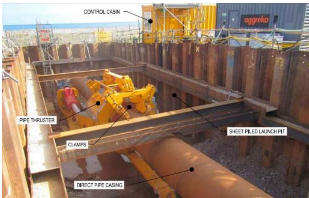
Figure 4.25: Direct Pipe Installation
