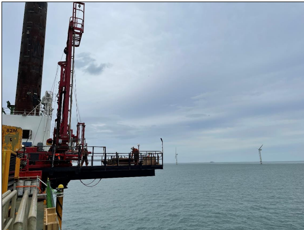
Figure 4.18: Borehole Drilling Rig at Arklow Bank
