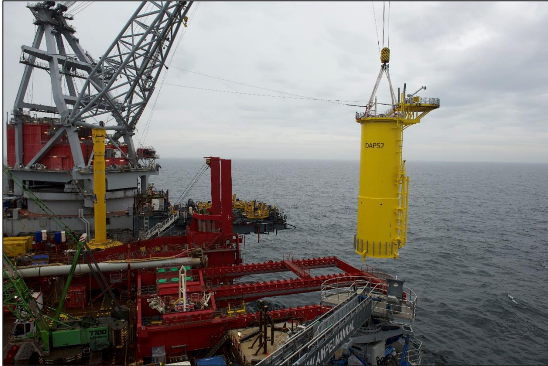
Figure 4.22: Offshore TP installation (Photo courtesy of Dogger Bank Windfarm)
